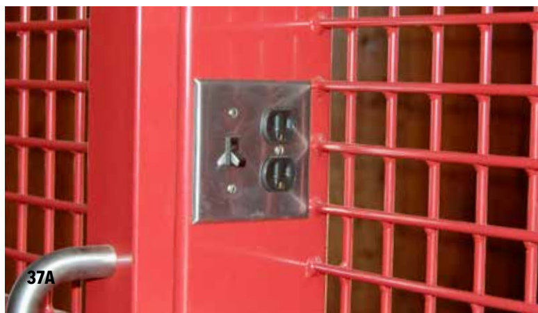
37A Electric outlets and switches can be integrated into your stall design, eliminating the unsightly conduit and increasing the safety of your barn.
